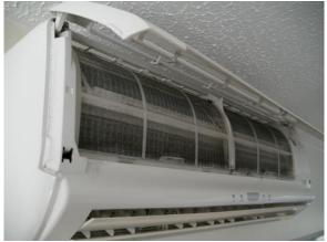
With the front of the heat pump cover lifted high, you can see the hinges. With a gentle pull the cover should slide out towards you.
